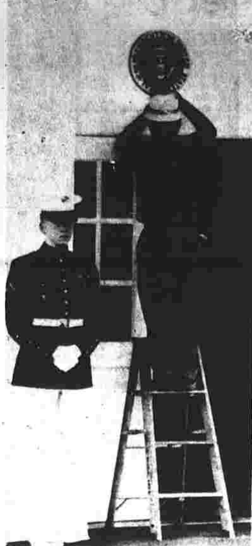
A workman installs a Presidential seal over the West Wing entrance to the White House, where for the first time it will hang. The seal along with Marine guard are recent Reagan Administration additions that have returned to the White House some of the trappings and formality that was discontinued by President Carter. (UPI photo)
